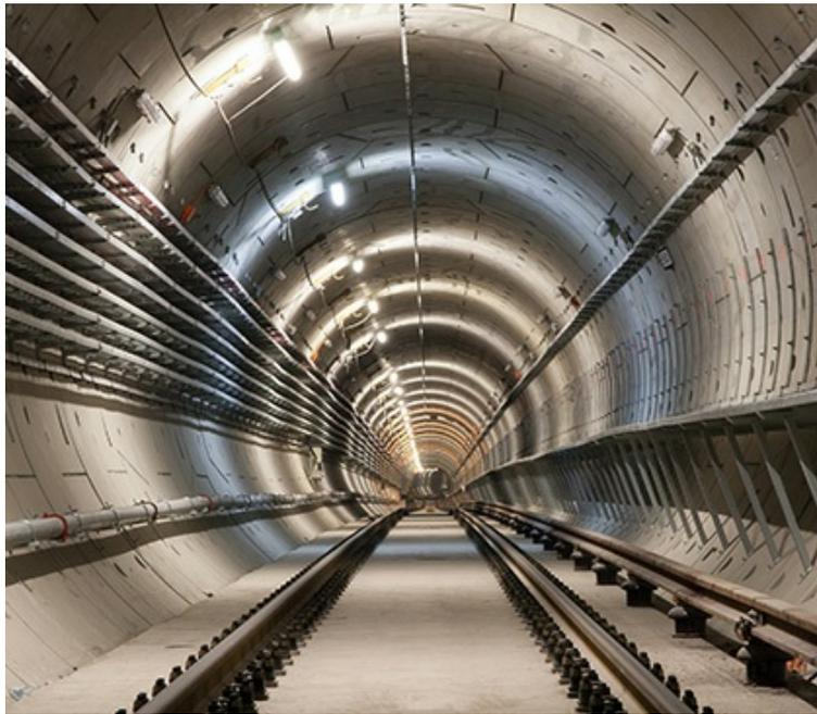
Four out of five winning transport business contractors chose Preprufe®Plus membrane based on its proven performance and the reputation of GCP Applied Technologies in the region. A fully bonded waterproofing membrane, this innovative system was installed before the concrete was poured and bonds to the structural concrete, preventing water tracking behind the waterproofing layer or problems caused by ground movements.
