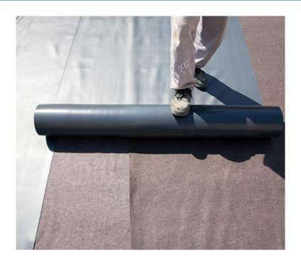
Due to its coastal proximity, museum construction structural engineers, SICA and Lamoureux & Riciotti, required a comprehensive waterproofing system, which would protect the slab from water ingress, provide protection from salt and sulfates in the ground and preserve the lifespan of the structure.
